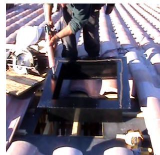
Figure 2 - Apply Sealant
