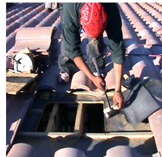
Figure 1 - Remove Battens
