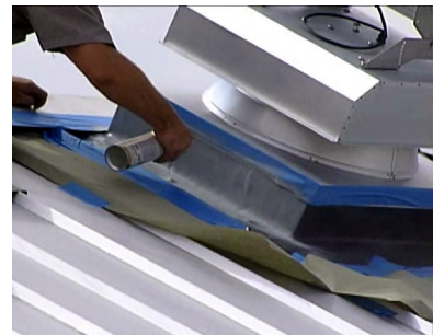
Figure 5 - Painting the Flashing
