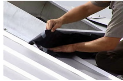
Figure 3 - Bottom Flashing
