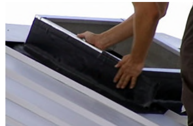
Figure 4 - Side Flashing
